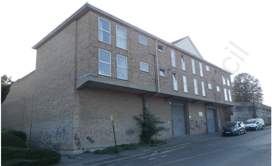
Figure 3: Photograph showing the front of Warren Hastings Court taken from Clifton Marin Parade.
