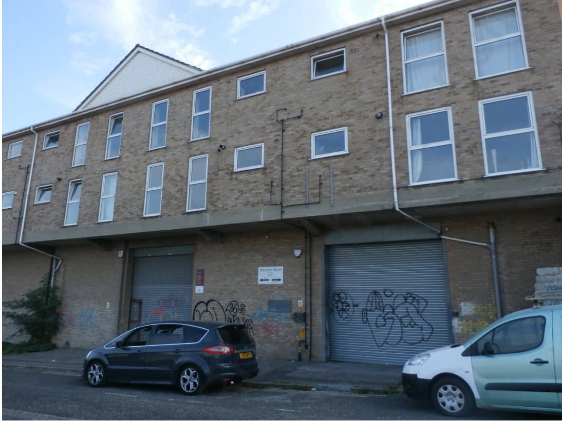
Figure 2: Photograph showing the front of Warren Hastings Court taken from Clifton Marine Parade.
