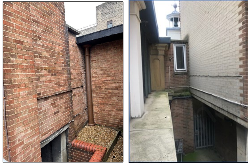
Figure 3: Views of the existing link, Image of left is looking south. Image on right looking north with RTP on the left.
