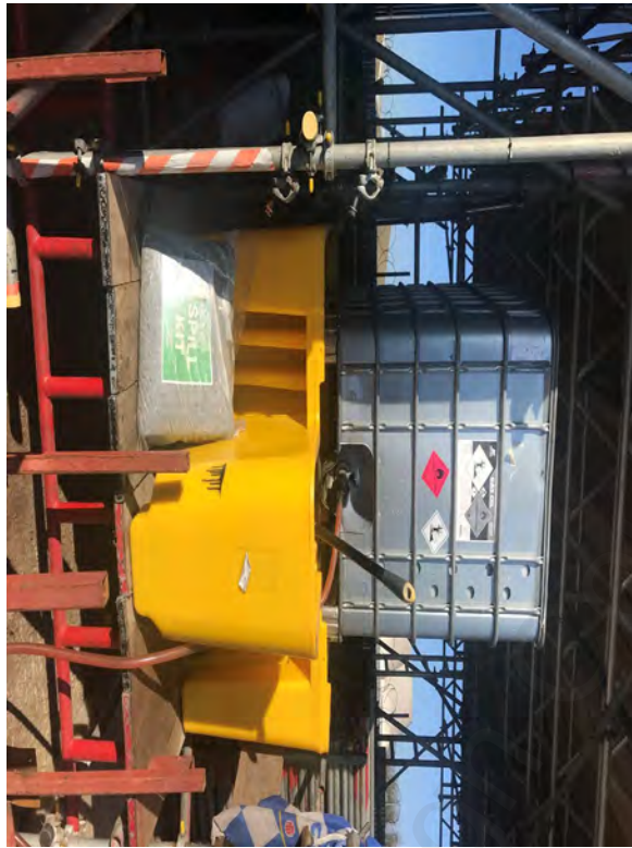
Photographic Plate No. 09: View of the 1000l above ground gas oil tank (bunded) with spill kit along the western boundary.
