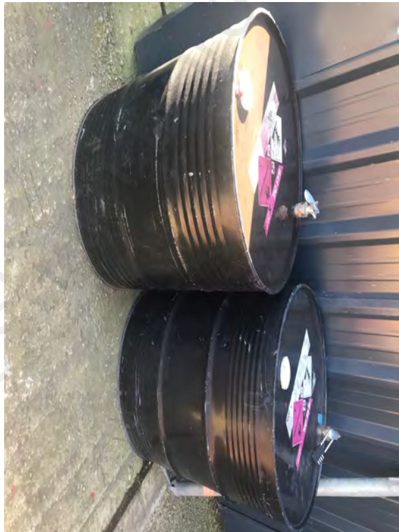
Photographic Plate No. 09: View of the 1000l above ground gas oil tank (bunded) with spill kit along the western boundary.
