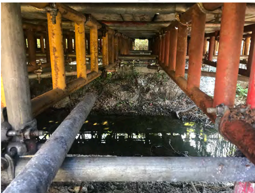
Photographic Plate No. 06: View of the surface water drain along the eastern boundary of the site.
