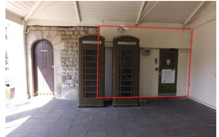
Connection between PCC and Pier – Pier undercroft
