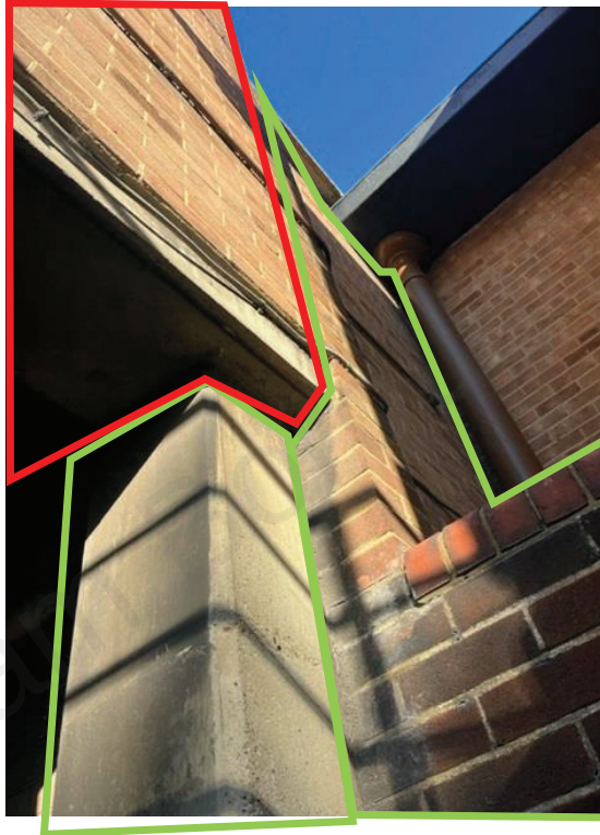
Connection between PCC and Pier – town side, hidden behind Pier
