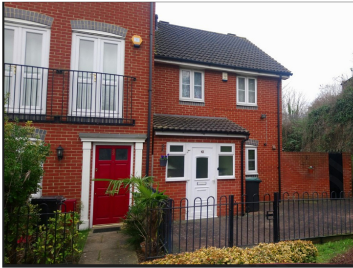
FRONT VIEW, HOUSE NO. 43 - 1, KENDALL GARDENS
