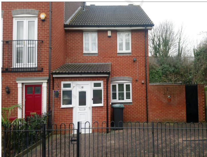
FRONT VIEW, HOUSE NO. 43 - 2, KENDALL GARDENS
