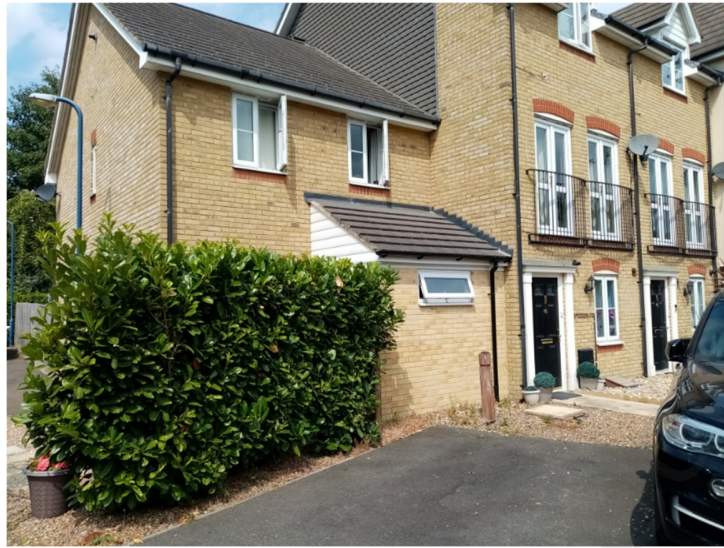
FRONT LEFT VIEW, HOUSE NO. 44 - 1, KENDALL GARDENS
