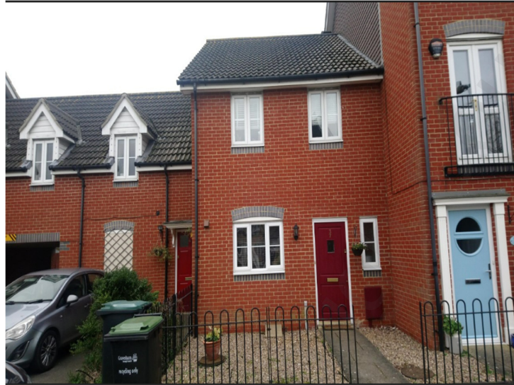
FRONT VIEW, HOUSE NO. 37 - 1, KENDALL GARDENS
