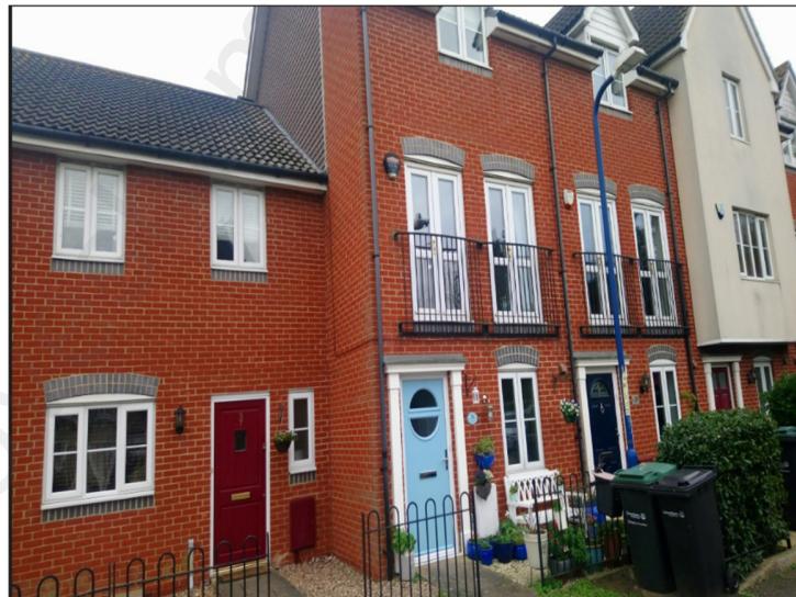
FRONT LEFT VIEW, HOUSE NO. 37 - 2, KENDALL GARDENS
