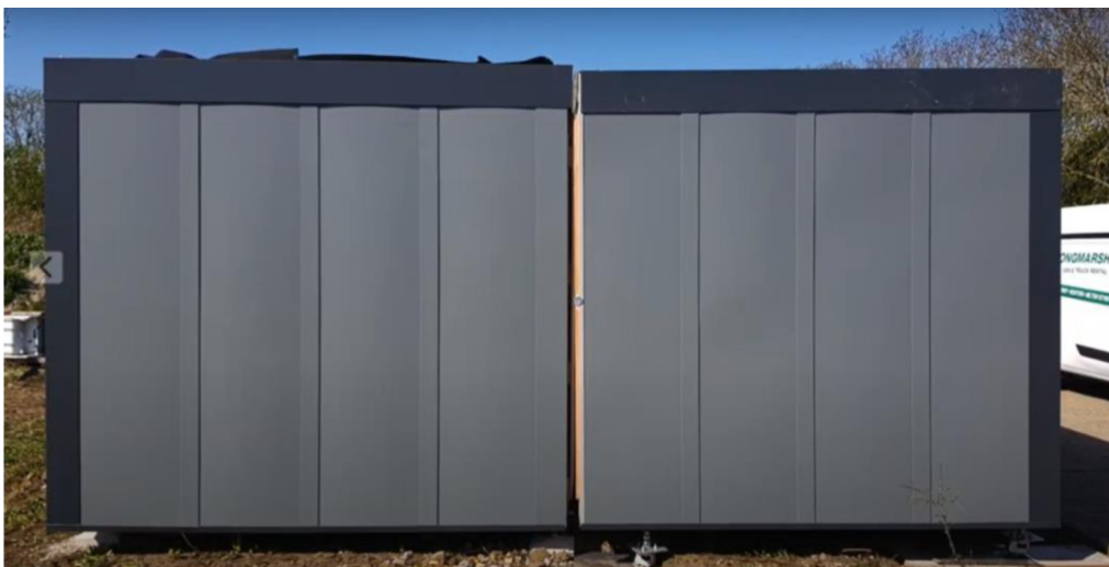
Second half in place just before it is rolled together and joined.
