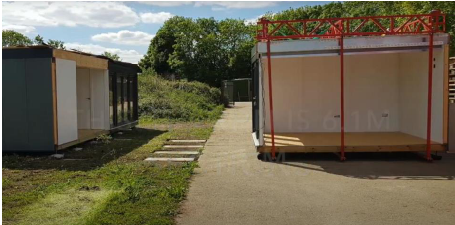
Second part of caravan within steel cradle for manoeuvring before joining
