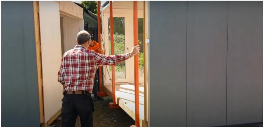
Second half being lifted into place on supporting cradle
