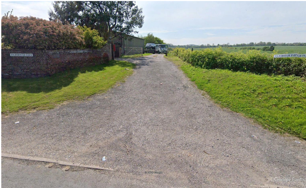
View from the Lower Higham Road towards the access drive. Just the side of the steel barn is visible as the barn is screened by existing walls and landscaping.
