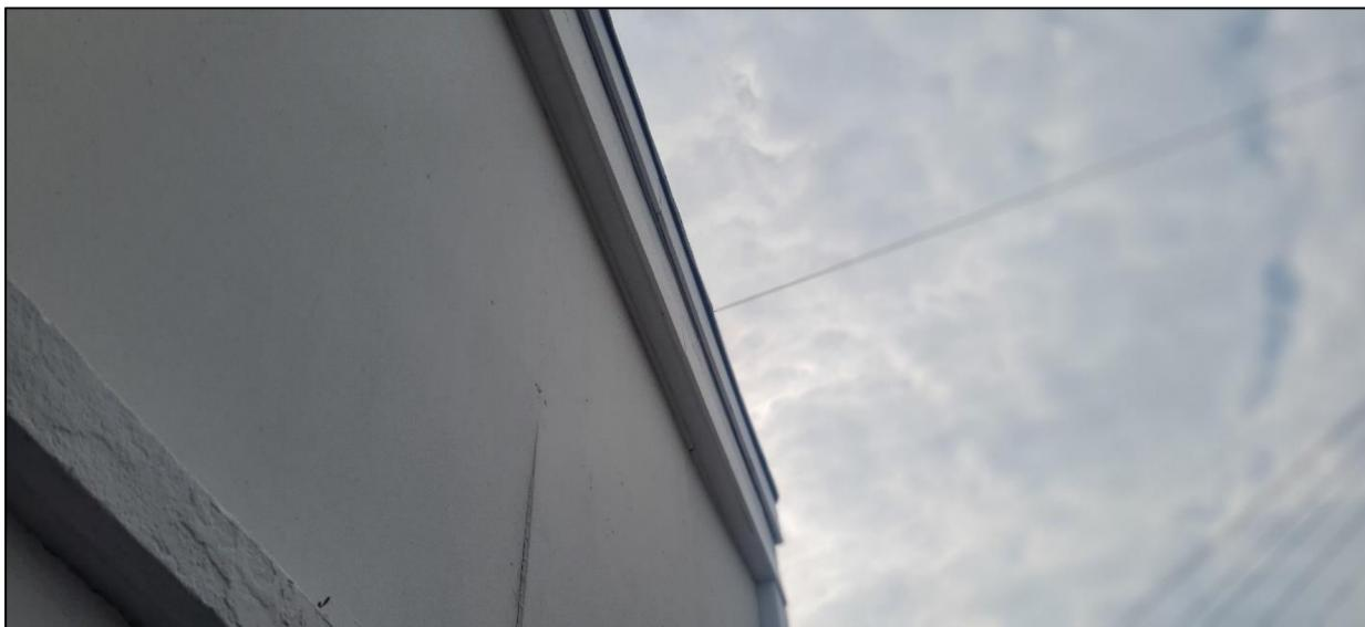
Photo 6: Small gap seen under fascia on southern elevation of B1.
