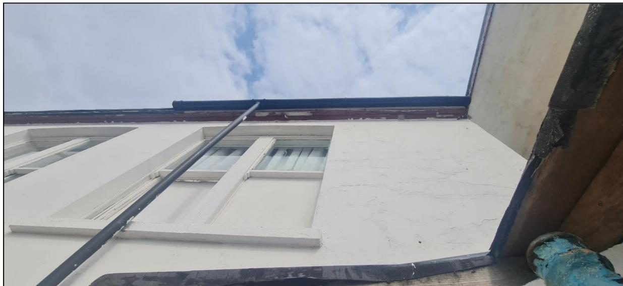
Photo 7: Small gap seen under fascia on eastern elevation of B1.
