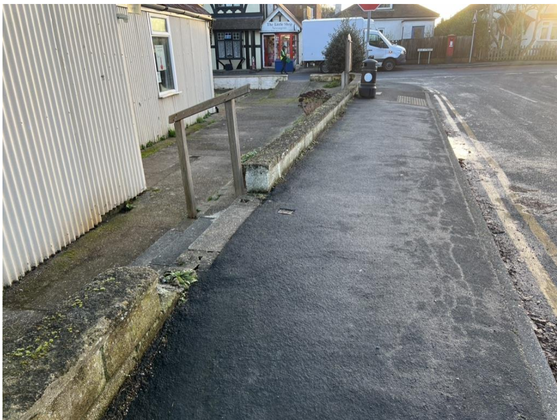
Photo (ii) – External paving and wall on Manor Road side
