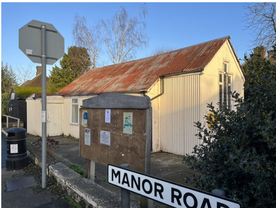
Photo (iv) – Existing elevation and boundary wall from Manor Road
