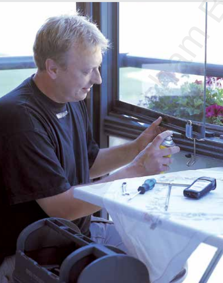
3 This first pane is turned inwards through 90°. Subsequent panes are then slid into the resulting space (opening position). As each pane is slid into the opening position, it can then be turned inwards. All panes can be turned inwards, providing a completely open balcony.
