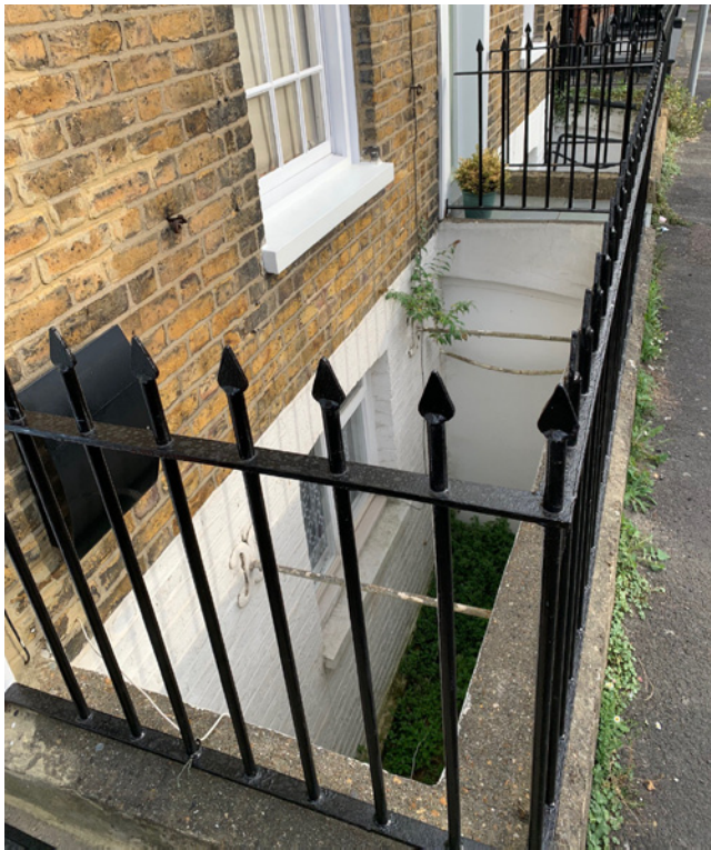
View of the existing lightwell
