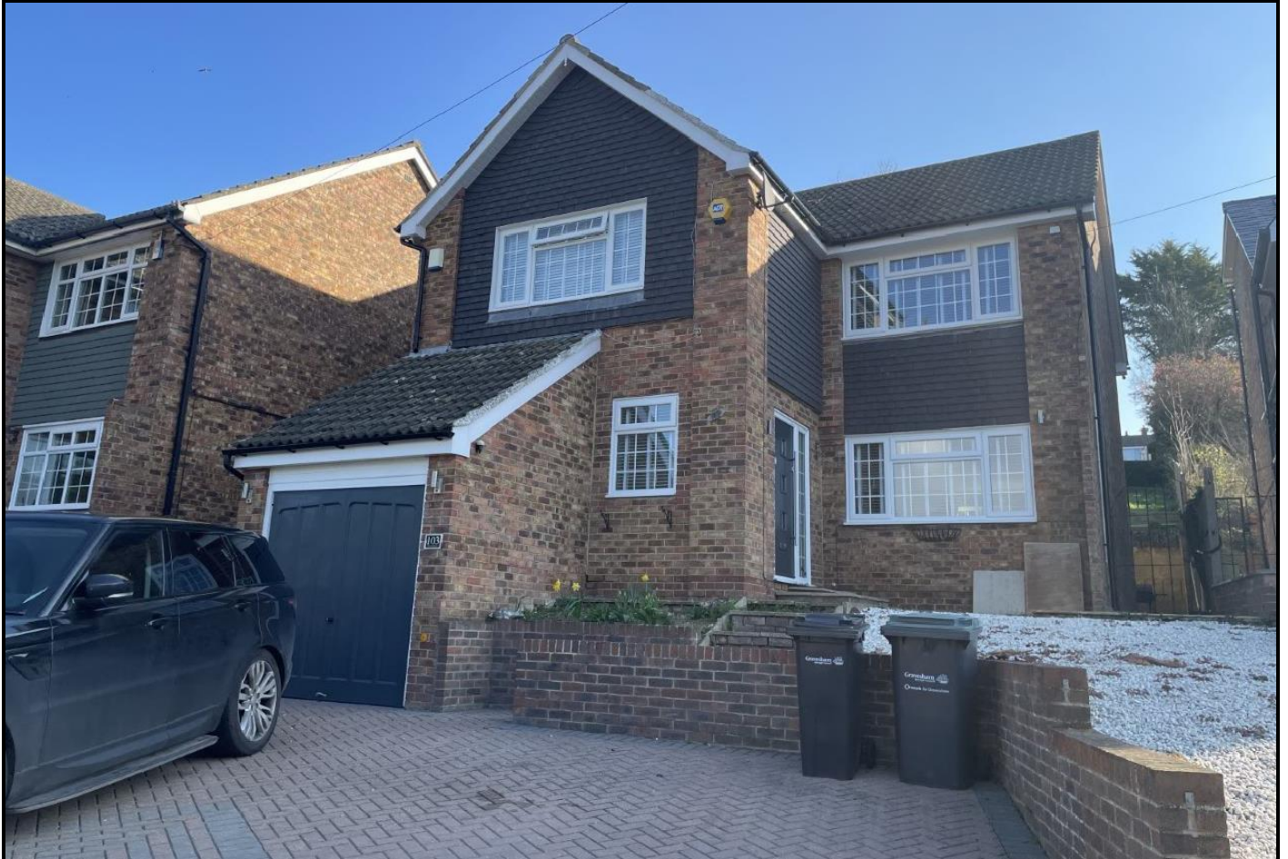
Image of Front Elevation taken during the site visit
