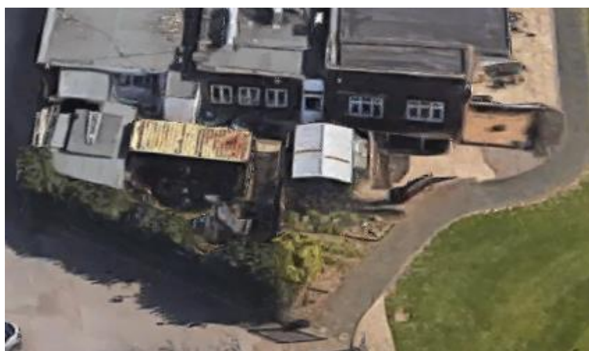
Google Image of western side of the clubhouse
