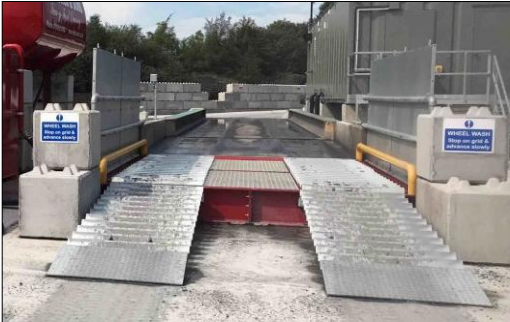
Figure 6.1 Example closed loop wheel wash
