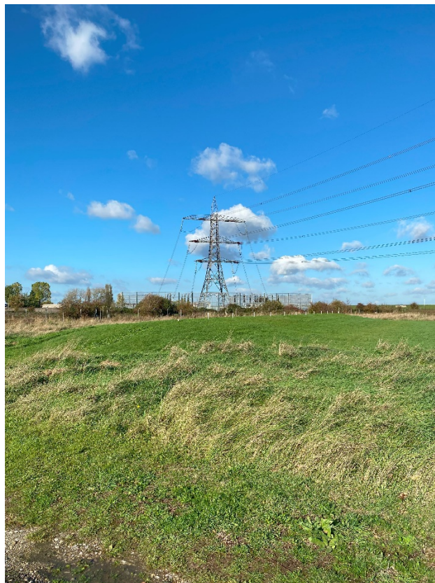
Photograph 10: South of the managed strip of the firing range looking back towards existing sealing end compound (November 2022)
