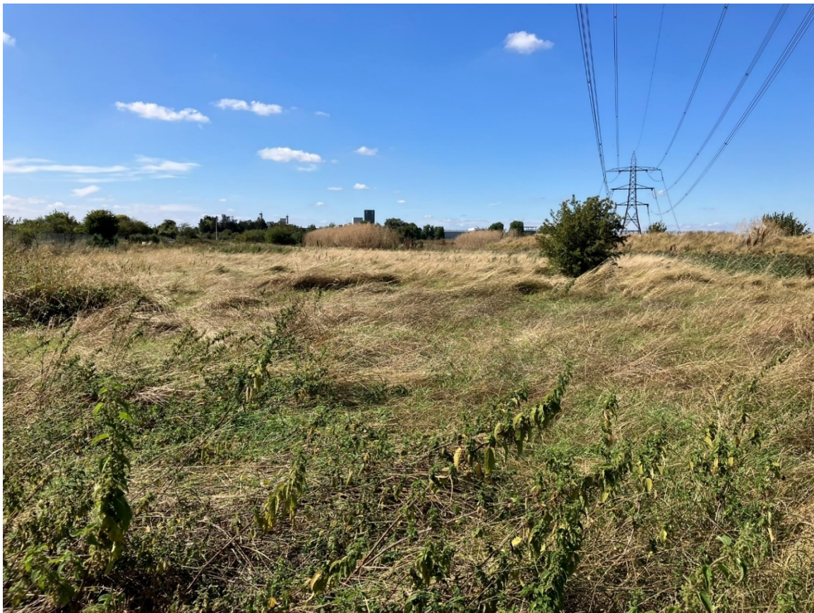
Photograph 12: Existing pylon route requiring grass cutting prior to restringing of overhead lines (late summer 2023)
