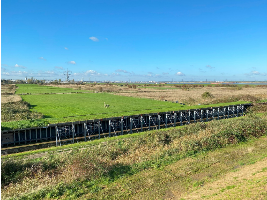
Photograph 11: Eastern end of the firing range looking west back towards Site (November 2022)
