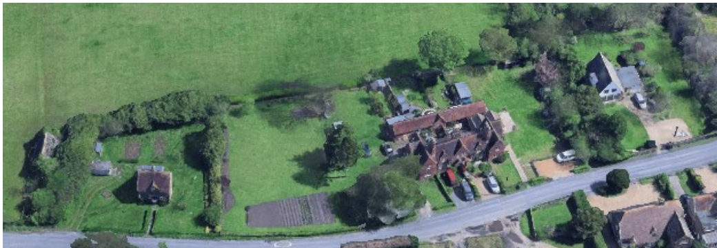
p-001 aerial view of site looking east
