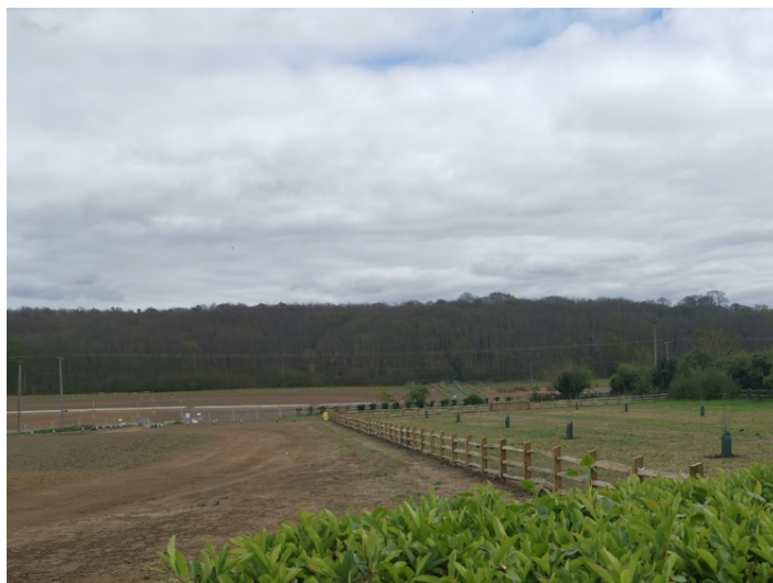
P-018 bio diversity works under construction to the east of the site.
