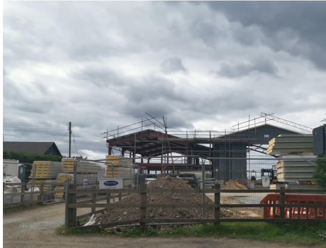
P-019 Storage units to west side of Thong Lane under construction
