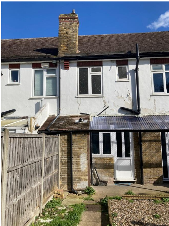
Photo Showing the Sewer Location & Manhole that is 2.8 Metres from the Rear Wall
