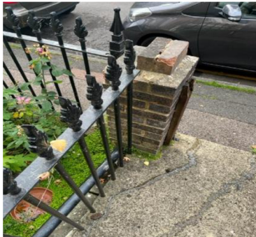
View of existing railings joining at corner with 28 Shrubby
