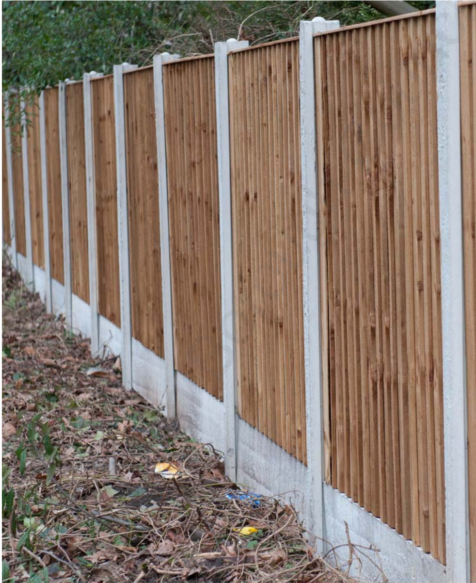
Close boarded timber fence with concrete post and base to match existing.
