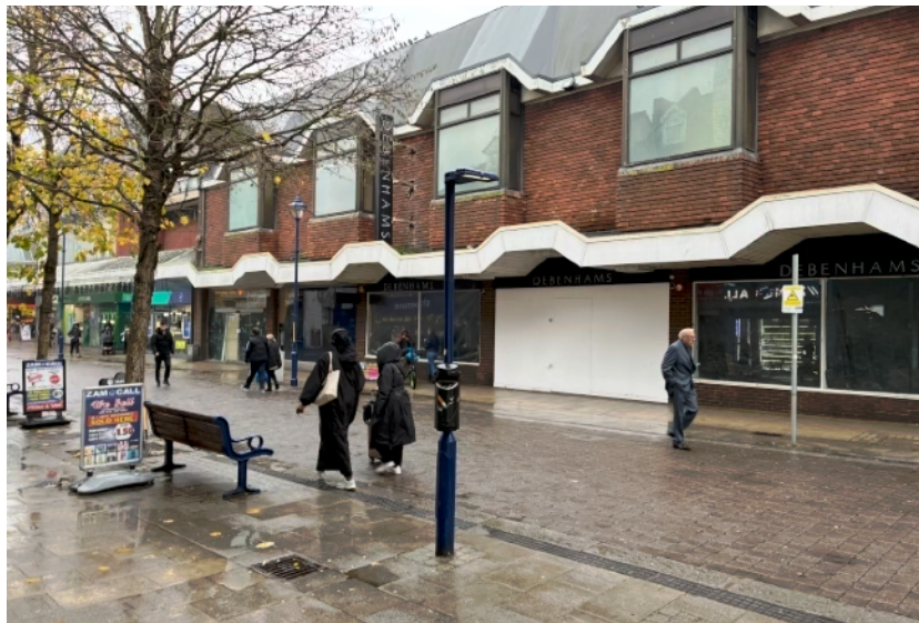
Figure 2: View from New Road
