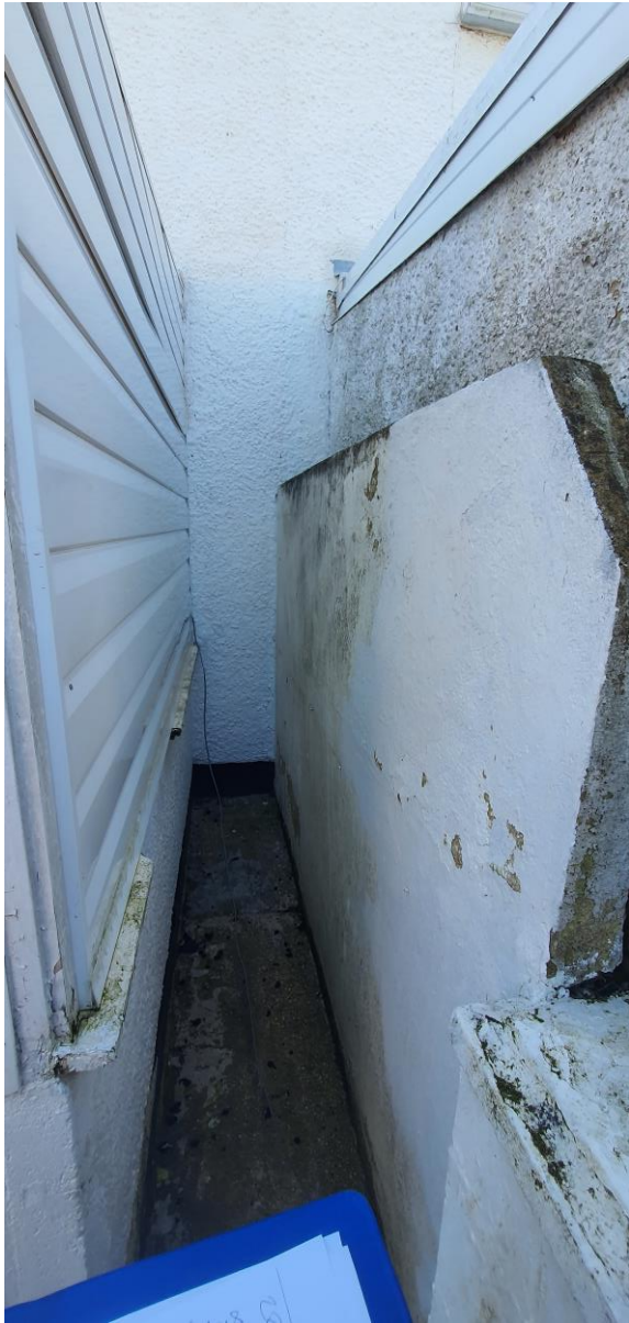
Gap between rear extensions
