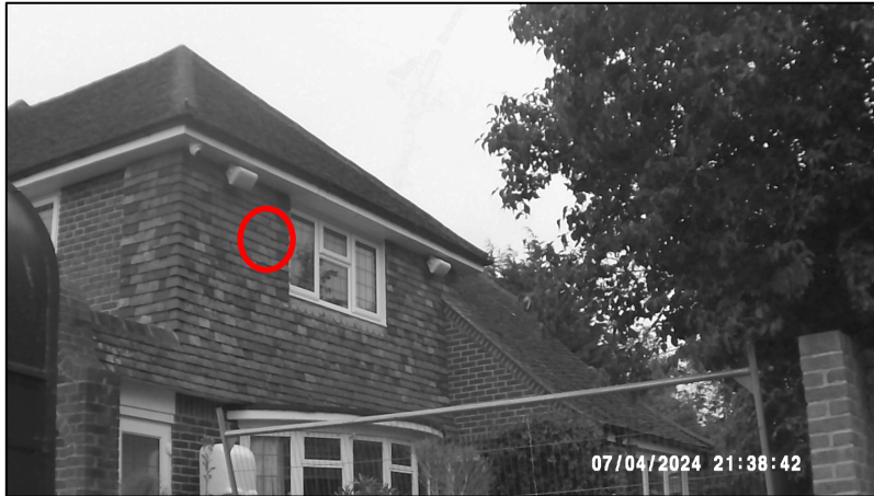
Figure 5 – 4 th July 2024 Common pipistrelle day roost on the south western elevation
