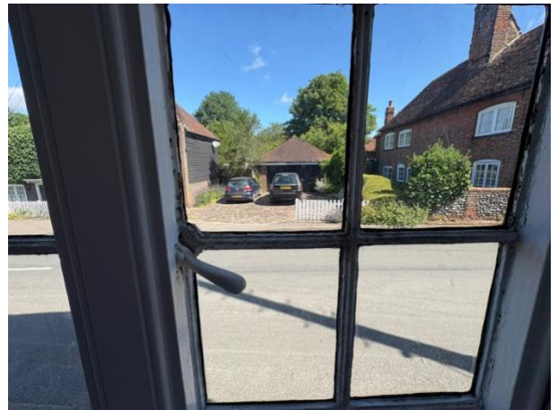
Figs 24-25: View of the existing cast-iron casements with timber frames at ground-floor level.
