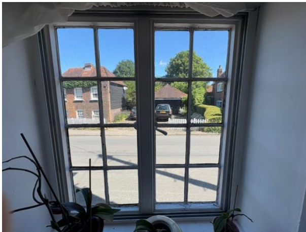
Figs 24-25: View of the existing cast-iron casements with timber frames at ground-floor level.
