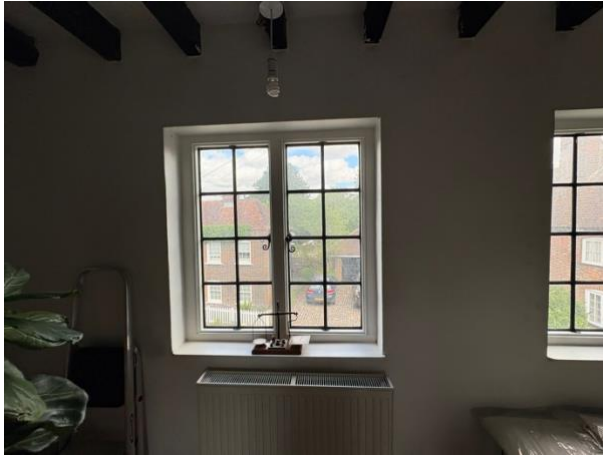
Fig 22: View of timber casements on first floor
