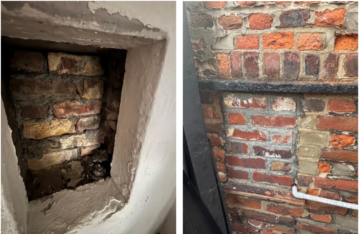
Figs 38 & 39: View of the existing infilled aperture.
