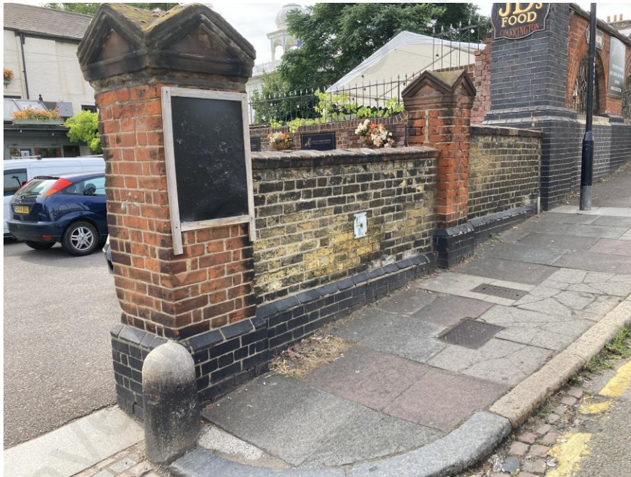
BOUNDARY WALL TO WELLINGTON STREET
