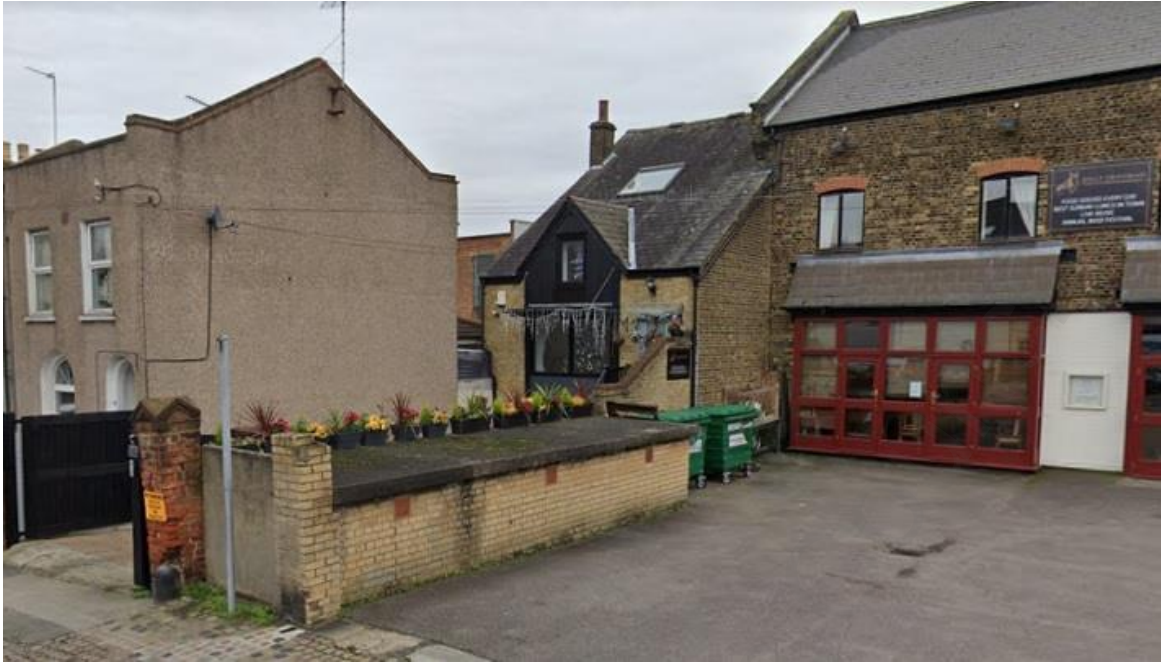
VIEW SHOWING STAIRCASE ENCLOSURE
