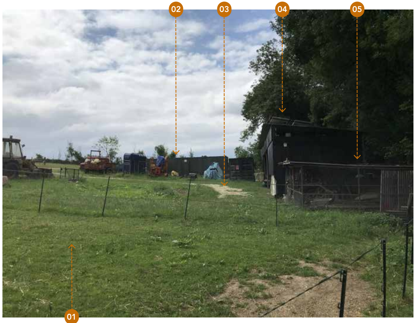
(Above) The barn shown on the right with surrounding structures and equipment to be consolidated.
