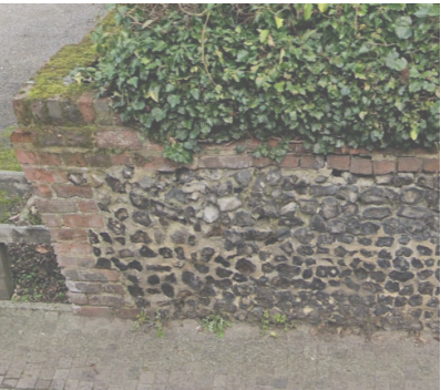
fence replaced with flint & brick wall
