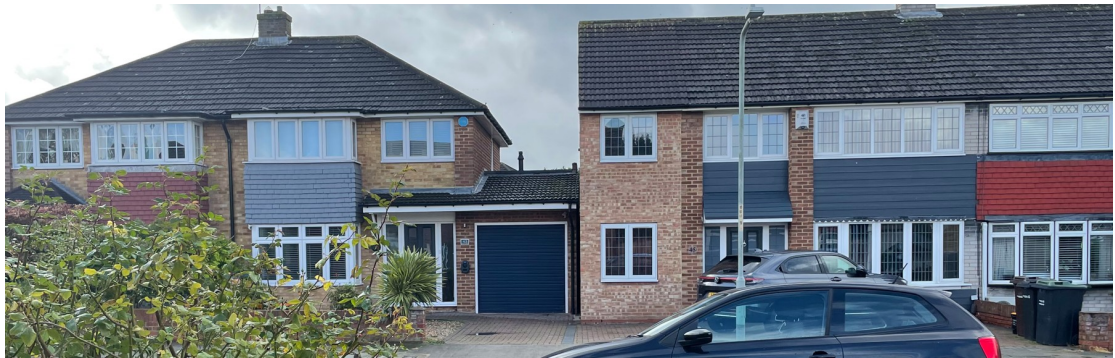
P – 004 opposite side of road we can see various differing treatments to hung tiles and cladding
