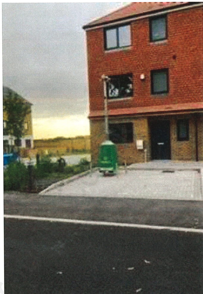
Parking & planking to No. 6
