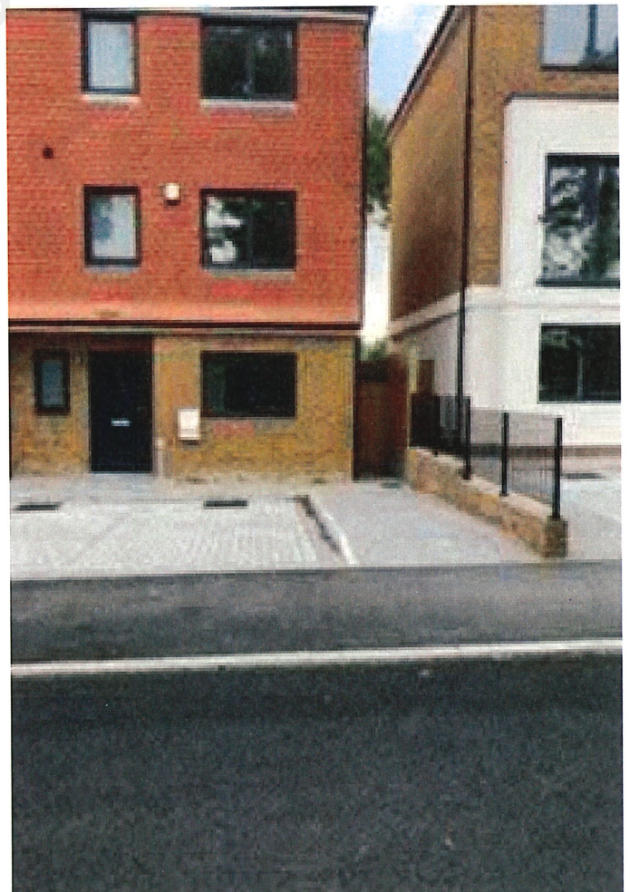
Paving, path + retaining wall in front of No 3
