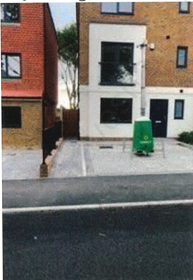
Retaining wall between nos 2 & 3
