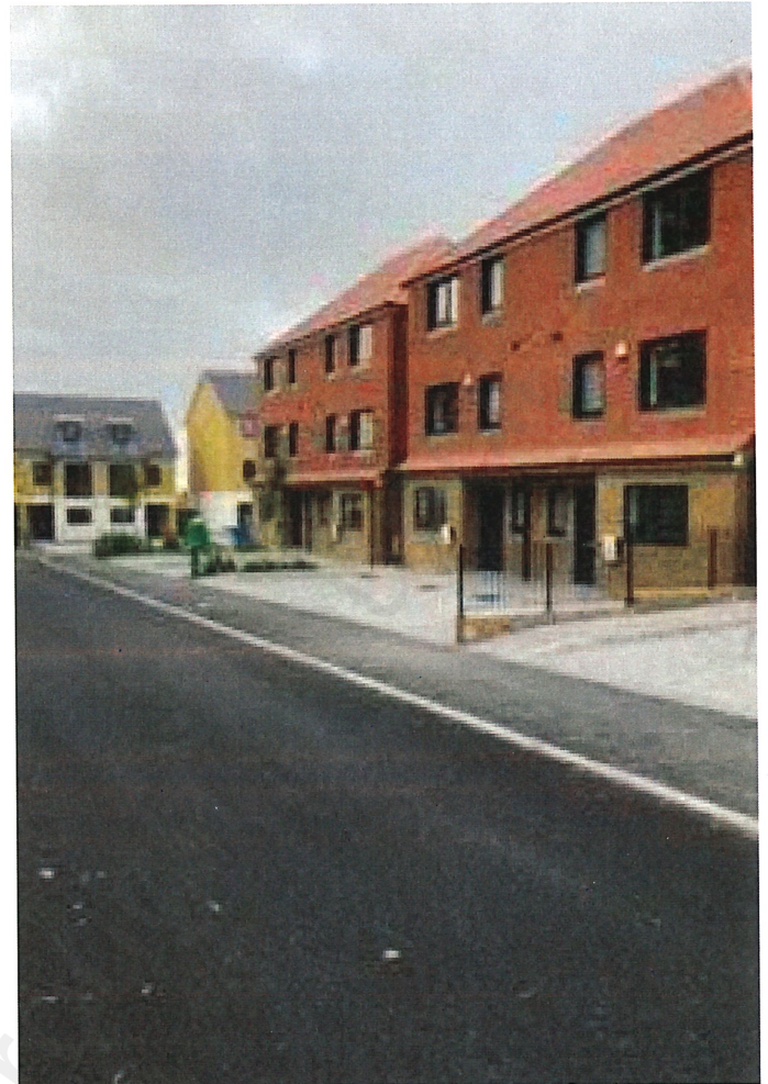
Paving, retaining wall + planting in front of Nos 3-6
