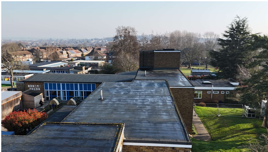
Image 2 – Roofs 2 & 3 note roof vents obstructions
