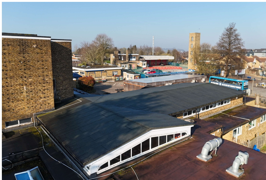
Image 2 – Roofs 2 & 3 note roof vents obstructions
