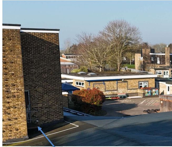
Image 15 – Metal Railings on Roof 1 access point
