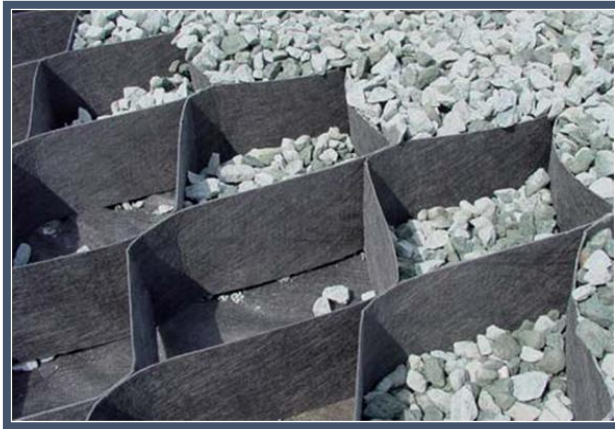
Figure 10 Examples of Cellweb filling with angular stone
