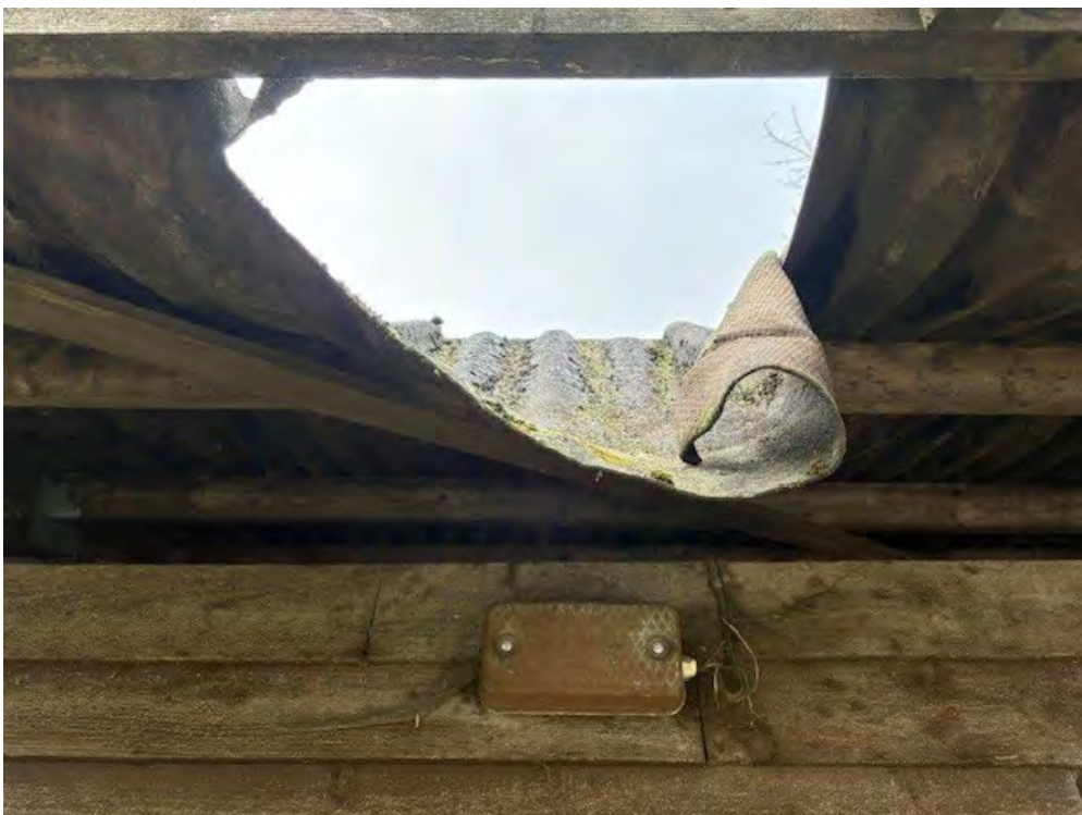
Plate 2: Stable roof with potential asbestos containing material (bitumen roof felt)
