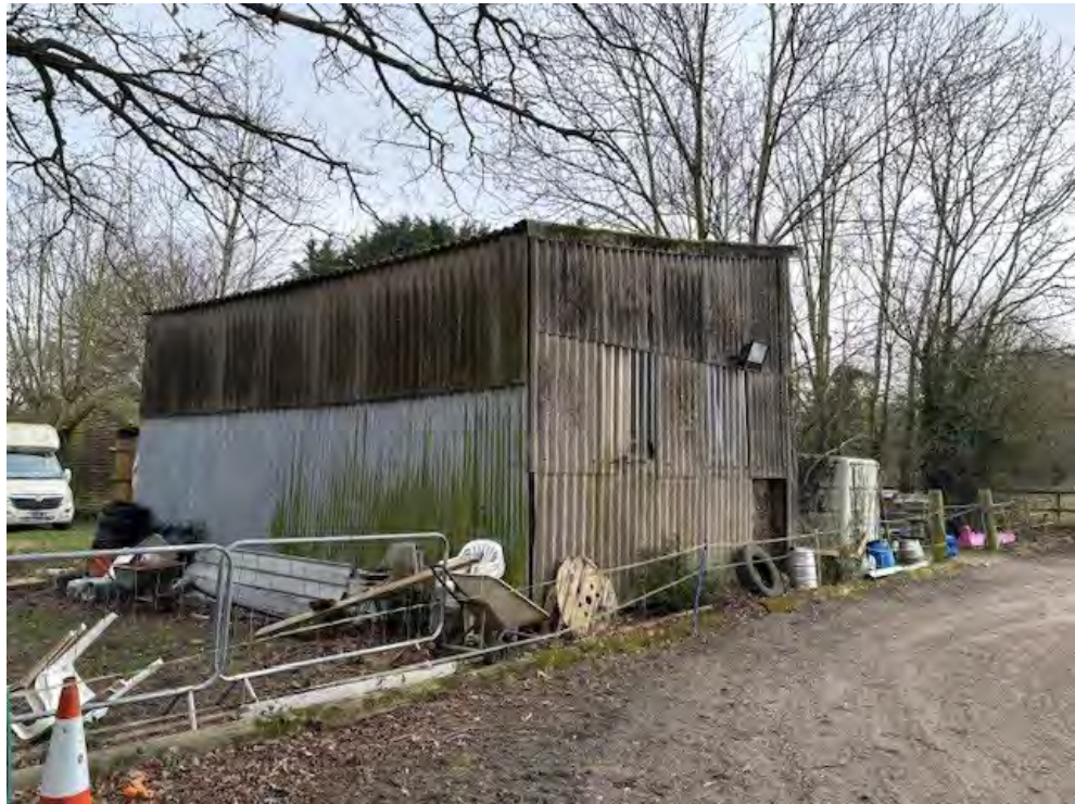
Plate 1: Shed with potential asbestos containing material (corrugated cement)
