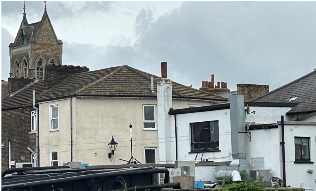
Figure 2- Measurement position showing microphone, kitchen extraction system and nearest receptor windows (Flat.204).
