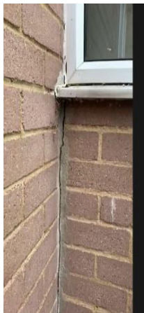
Picture 1: Left side of porch
