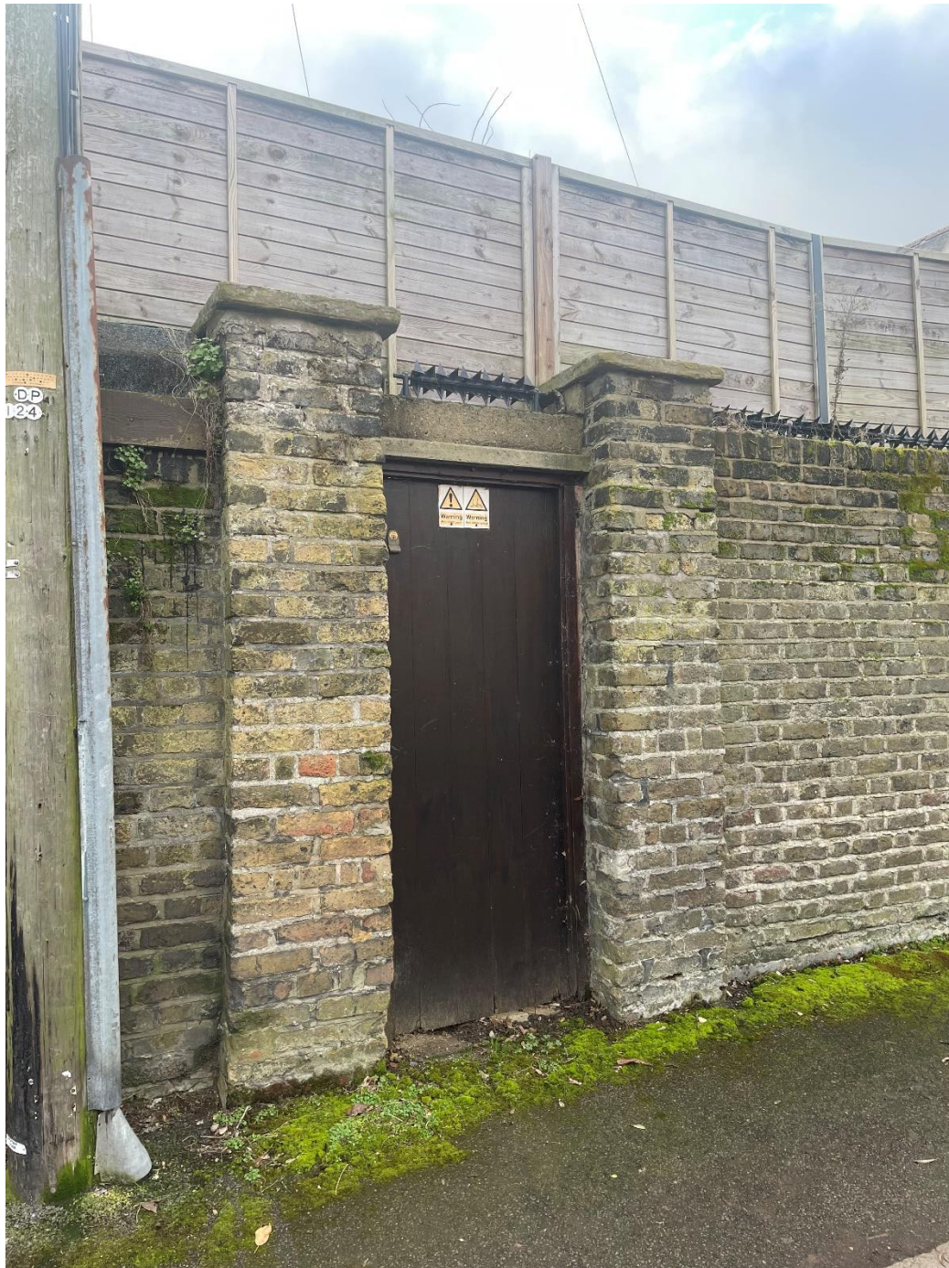
Fig.04 – Street View from William Street, pedestrian access
