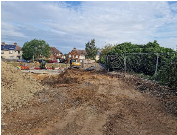
Figure 1. Area where G5 needs to be removed in relation to the new sub-station is comprised of Ivy and 1no. elder.
