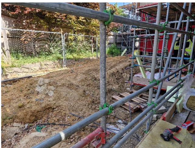
Figure 1. Area between T01 and ongoing construction works.
