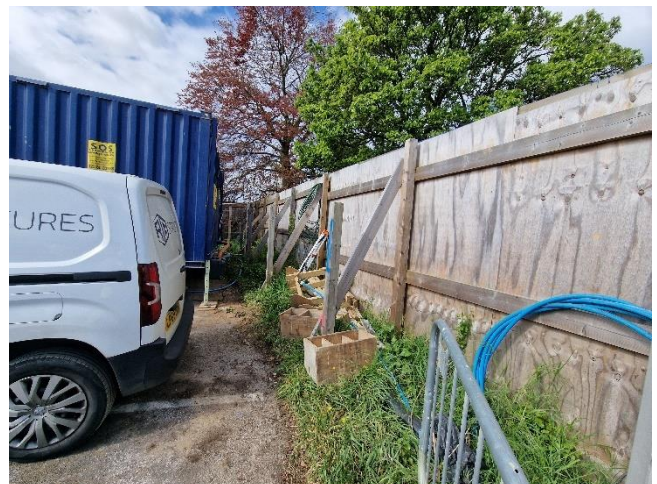
Figure 6. Existing hard standing, site hoarding, temporary office in relation to the TPO beech tree (T1) and pear tree (T2).
