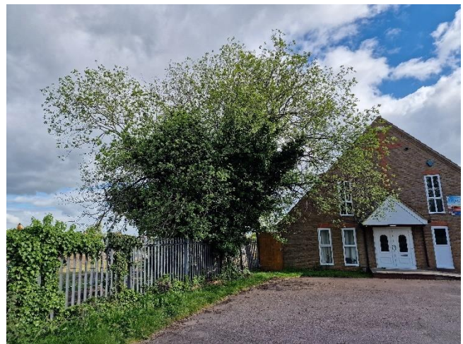
Figure 2. Goat willow (T10) to the south in conflict with the fence.
