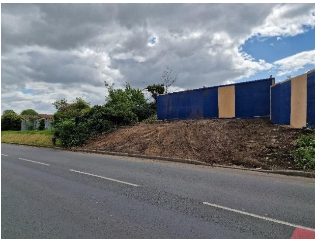
Figure 1. Location of northern access, and part removal of G3.
