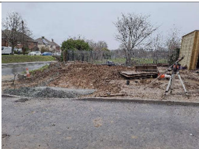
2. Looking northeast, outstanding landscaping work remains at the site entrance.
