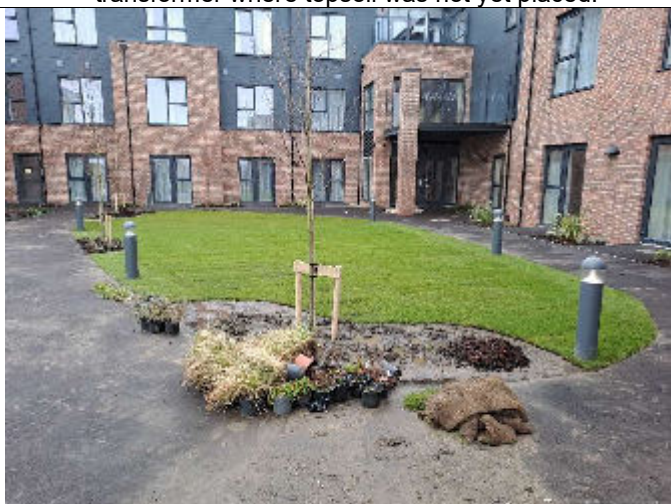
4. Looking west, the grass turfed roll being placed in the area behind the building.
