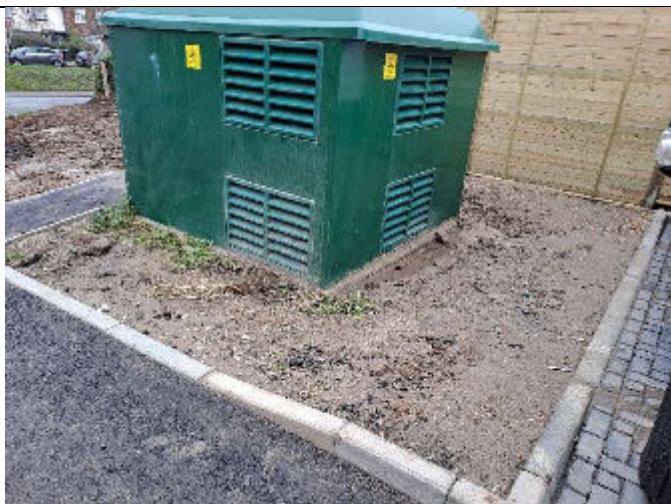
2. Looking northwest, the area surrounding electrical transformer where topsoil was not yet placed.
