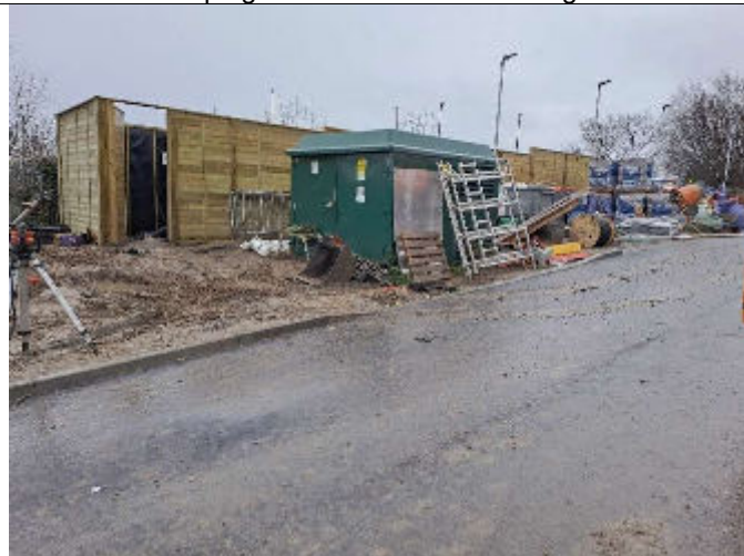
3. Looking northeast, incomplete topsoil placement near the site entrance.
