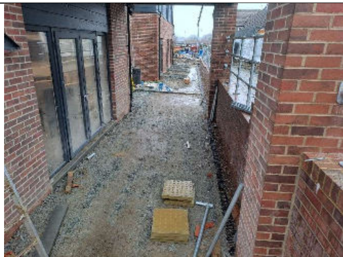
5. Looking northeast, ongoing topsoil placement along the side of the building.
