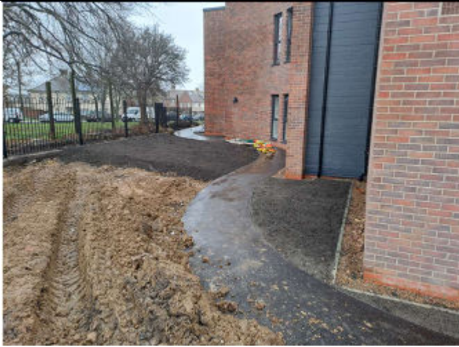
7. Looking northeast, ongoing topsoil placement along the northern perimeter fence
