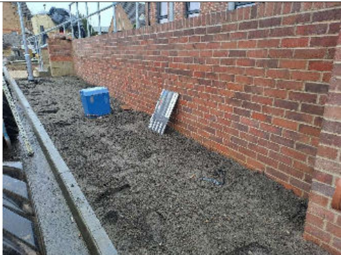
4. Looking southeast, topsoil placement at the front of building.
