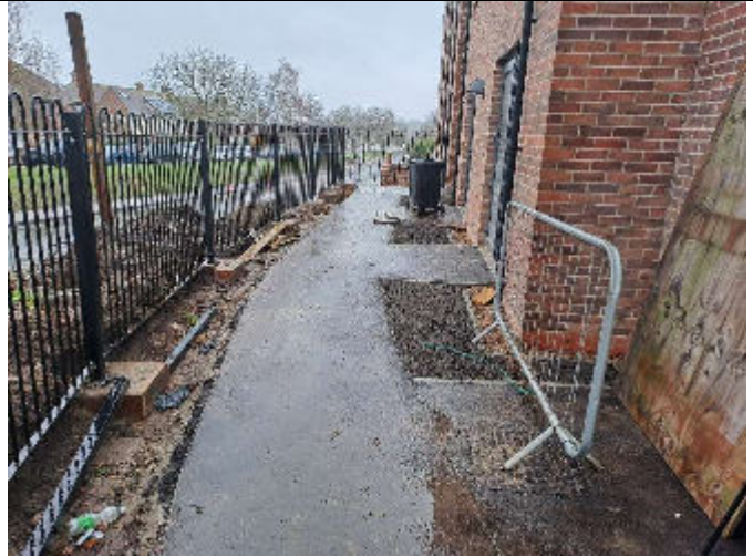
8. Looking northeast, topsoil placement next to the building and the perimeter fence.
