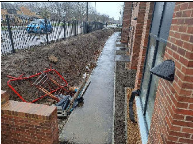
6. Looking northeast, ongoing topsoil placement along the side of the building and the perimeter fence.
