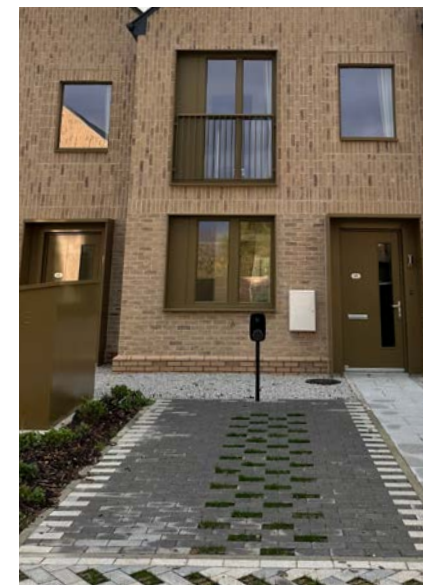
Fig. 5.33. EV charging point
