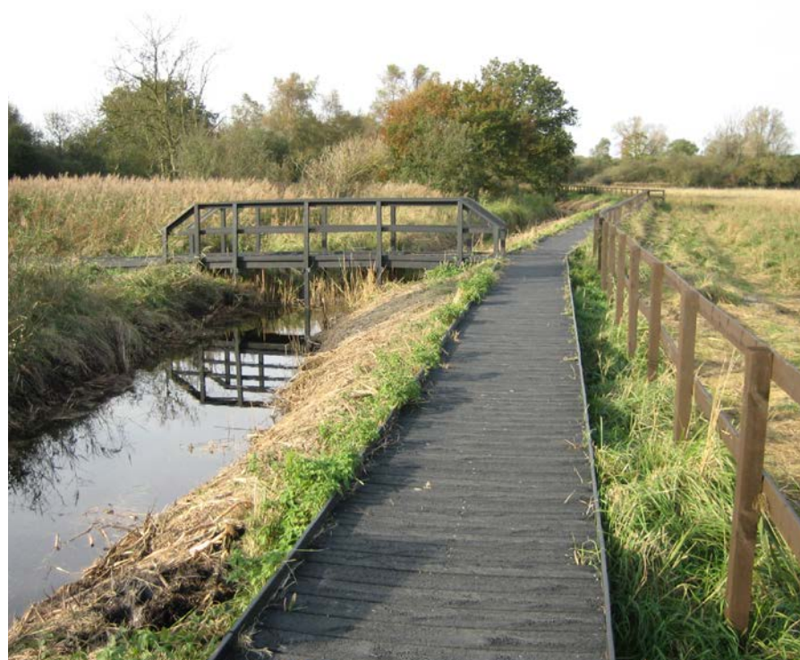
Fig. 5.24. Boardwalk over water basin
