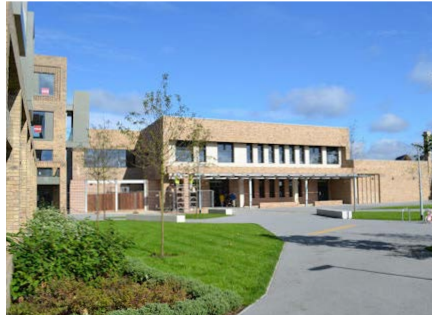
Fig. 5.27. Trumpington Meadows Primary Schools - main building and frontage integrated with the surrounding urban form and public realm.
