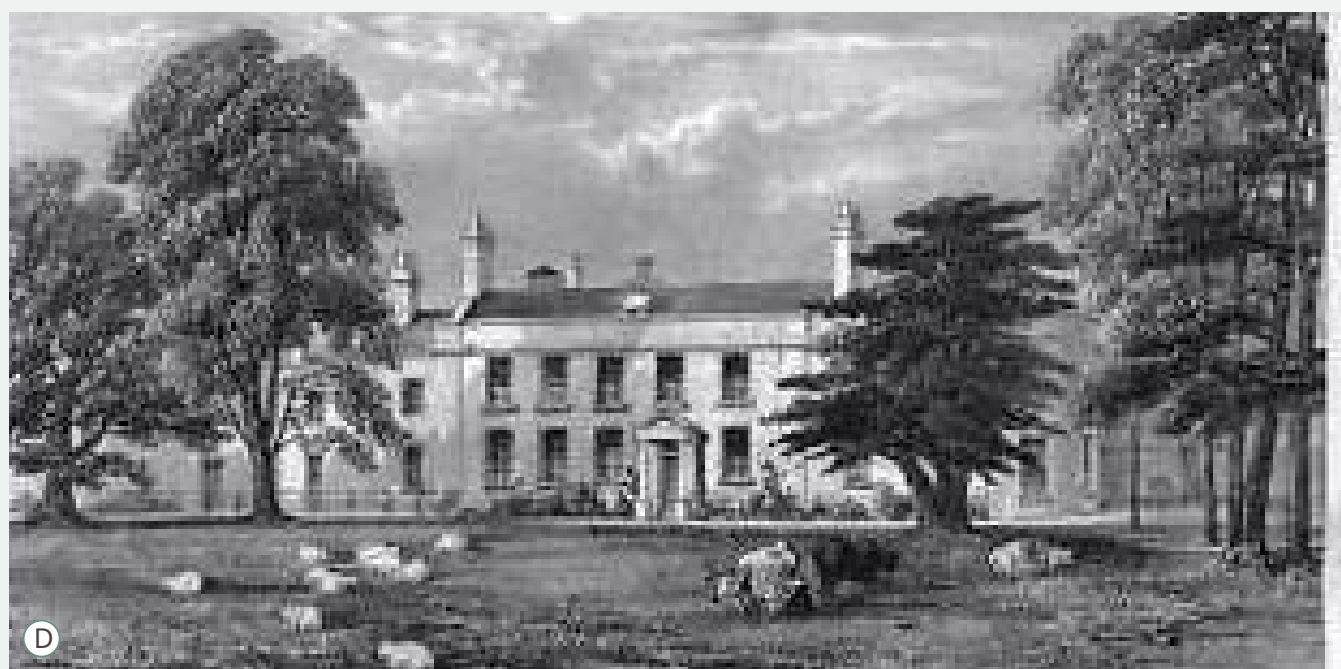
Fig. 3.26. Camer House C. 1838
