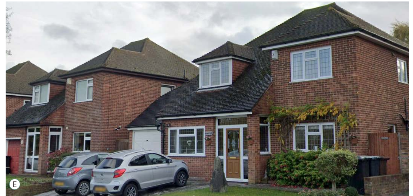
Fig. 3.41. Typical contemporary housing in Sole Street
