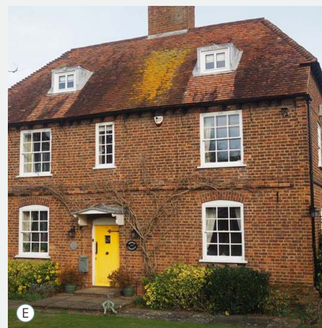
Fig. 3.27. Norwood Farmhouse (Grade II)
