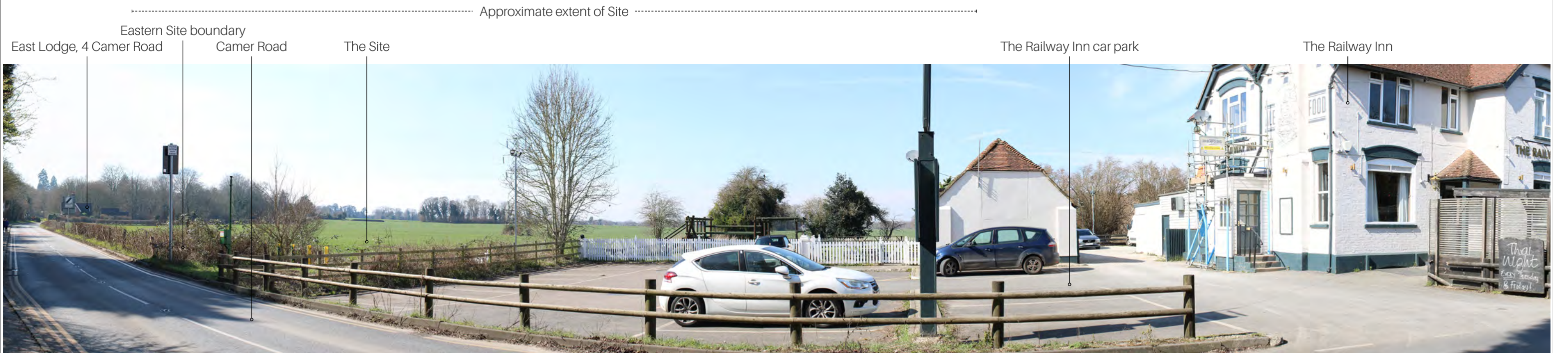
Photograph no. 16b Winter 2025 - View west towards Site from Camer Road.
