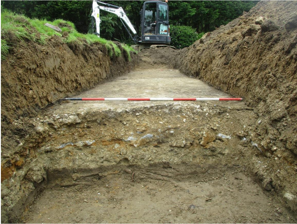
Plate 5. The concrete road/hard-standing and its underlying levelling/consolidation (two-metre scale, looking south-east-south)
