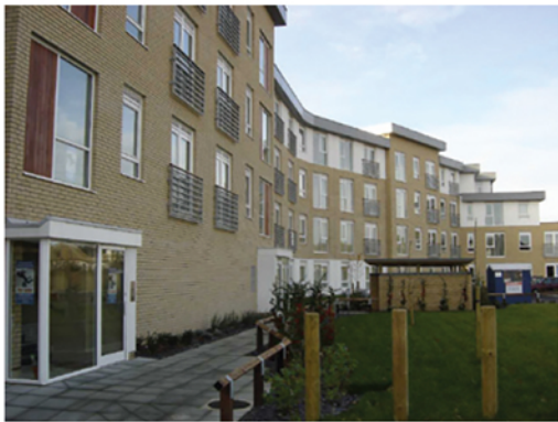
[2] Windows & External Doors Comar 5P.i ECO+ ([2a] Windows- White, [2b] External Doors- RAL 7013- Brown Grey*) * to coordinate with zinc cladding
