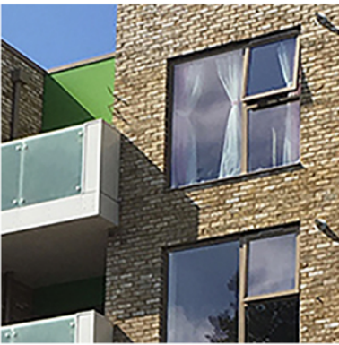
[2] Windows & External Doors Comar 5P.i ECO+ ([2a] Windows- White, [2b] External Doors- RAL 7013- Brown Grey)
