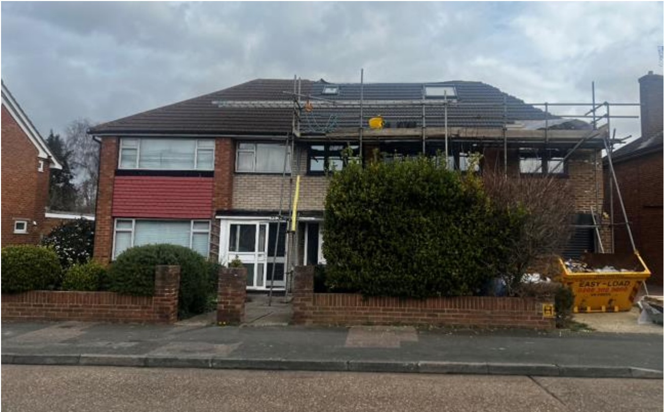
Extension at No.96 Vigilant Way.
