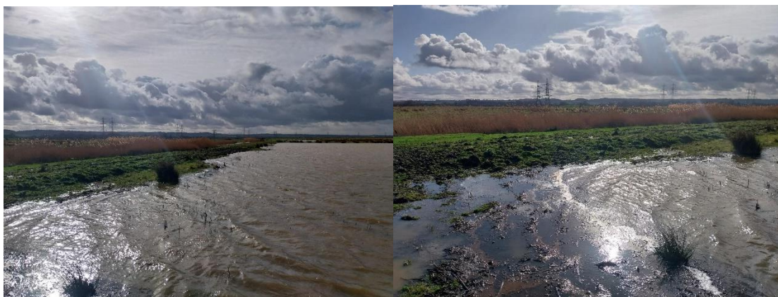
Figure 4: Bund installed at RSPB Higham Marshes, adjacent to Shorne Marshes, in December 2022 planning granted by Gravesham Council. (20220575). Image: RSPB
