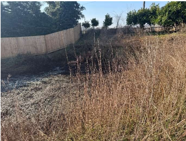
Print 7 View of front embankment
