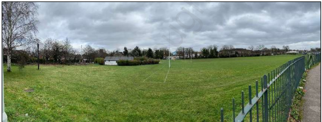
Above: View of existing Bowls Pavilion and sports pitches to the south
