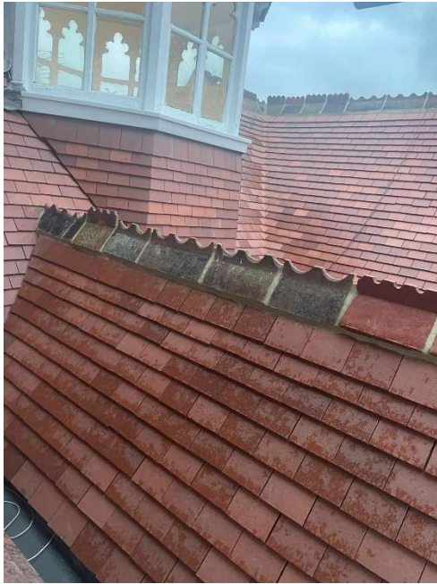
Previously Installed Tile – Image 3
