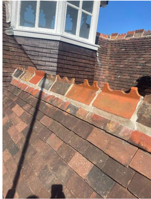
Newly Installed Tile – Image 3
