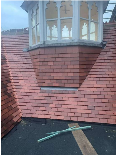
Previously Installed Tile – Image 1
