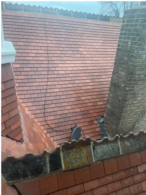
Previously Installed Tile – Image 2
