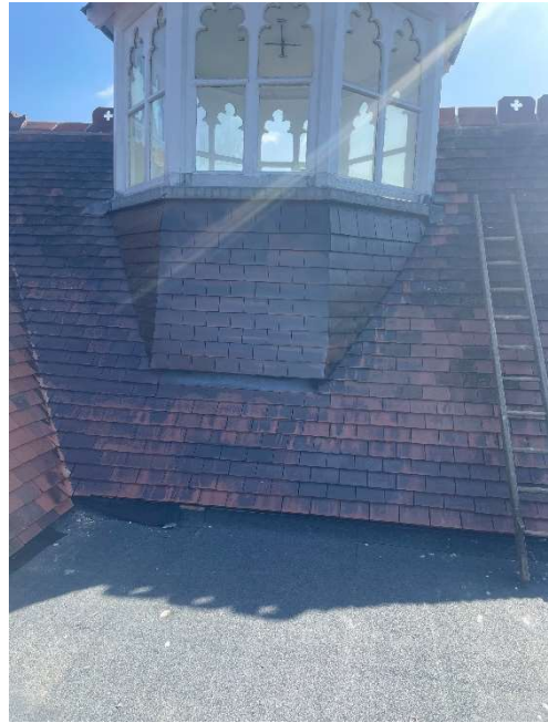
Newly Installed Tile – Image 1
