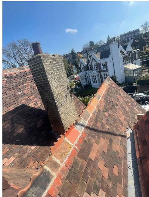
Newly Installed Tile – Image 4
