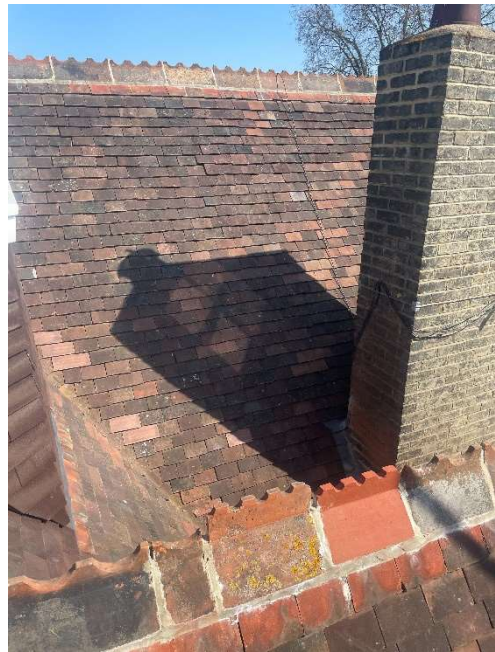
Newly Installed Tile – Image 2
