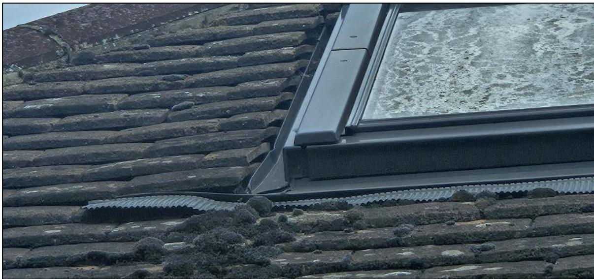
Photo 6: Loose tiles on the western elevation of B1.
