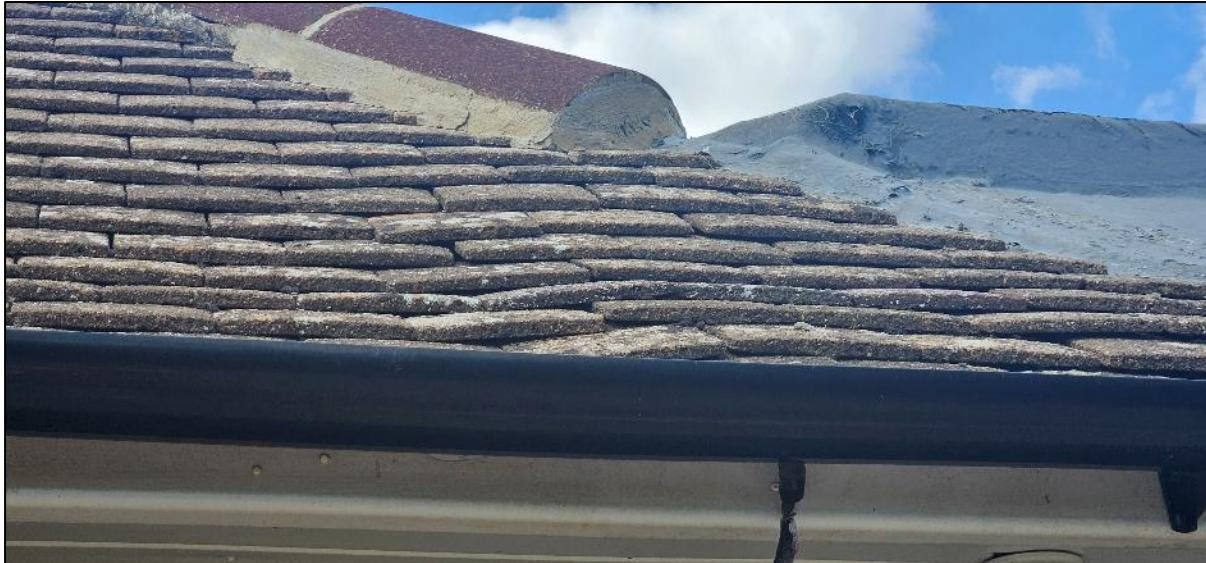
Photo 5: Loose tiles on the southern elevation of B1.
